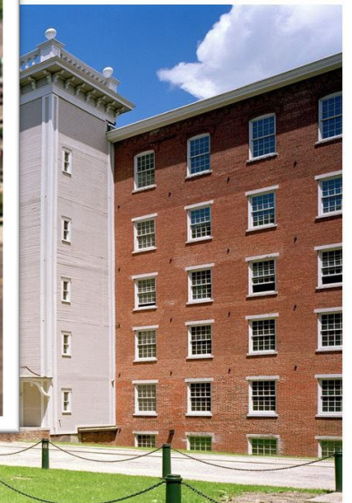
In Lowell, Massachusetts, the textile industry is gone, but the mills that gave the city its identity remain, now repurposed as housing, offices, retail and other uses. Photo courtesy of Ed McMahon
